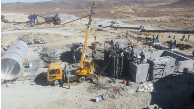
Foundation and structure
